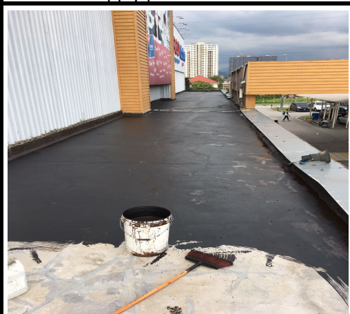
Photo 6 Applying of primer
