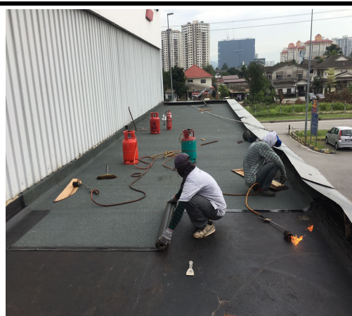
Photo 5 Torch on membrane work
