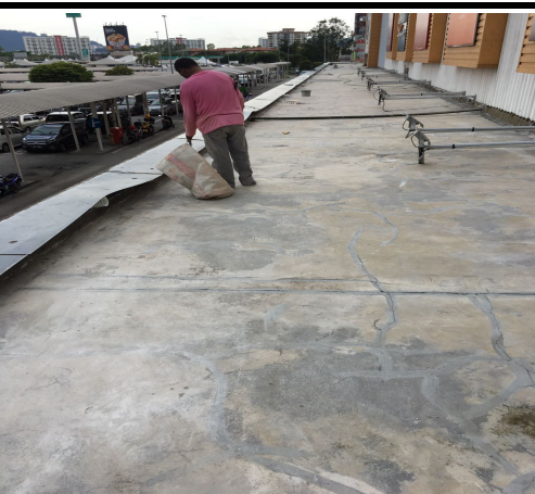
Photo 5 Cleaning before apply primer
