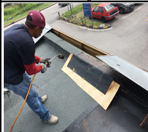
Photo 12 Torch-on membrane
