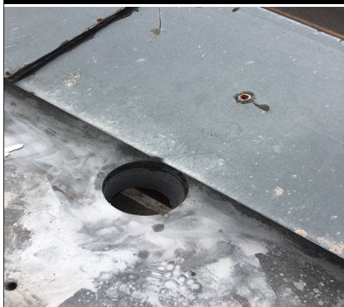
Photo 4 Coring 6"- install downpipe
