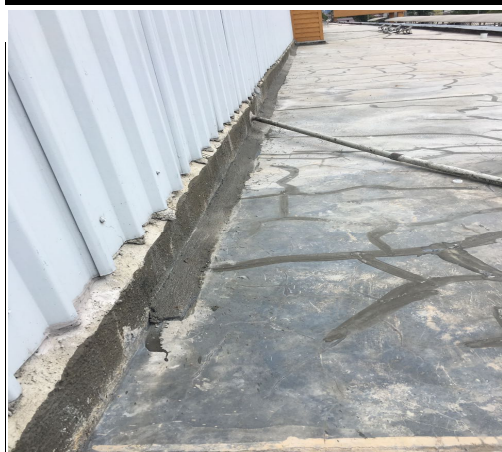
Photo 1 Angle fillet at all corner
