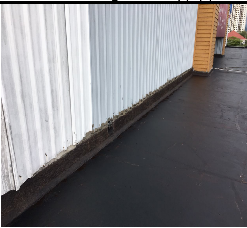
Photo 8 Primer application view
