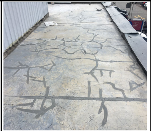
Photo 12 Crack repair
