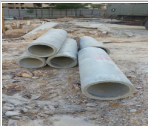
RC culvert pipe unload Photo 4
