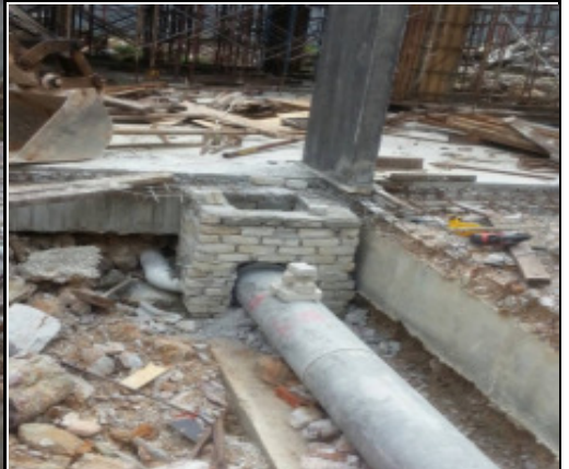
RC culvert pipe installation WIP. Photo 3
