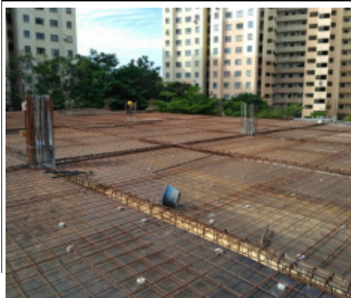
Photo 7 1 st layer BRC installation complete.
