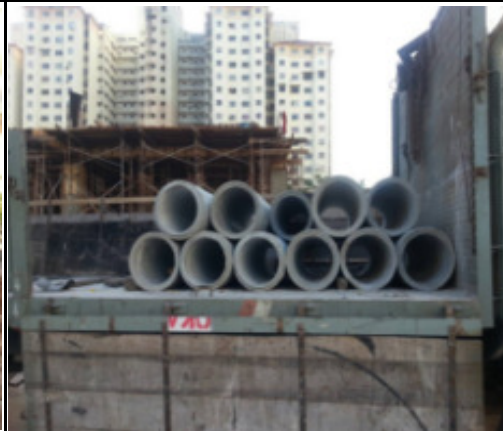
RC culvert pipe arrived at site Photo 2
