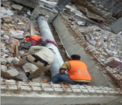
RC culvert pipe installation WIP. Photo 1
