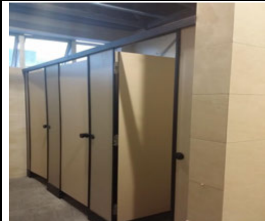
Photo 8 Male Toilet Cubicle completion
