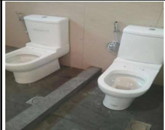
Photo 9 WC installation view
