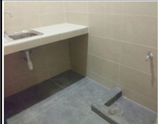
Photo 6 Pantry c/w ablution area...
