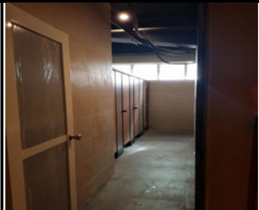
Photo 6 Female Toilet cubicle view
