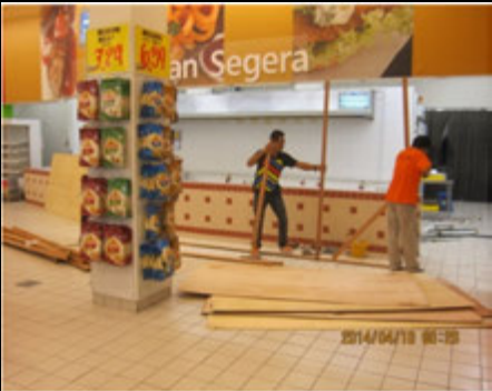
Photo 1 Material store room
