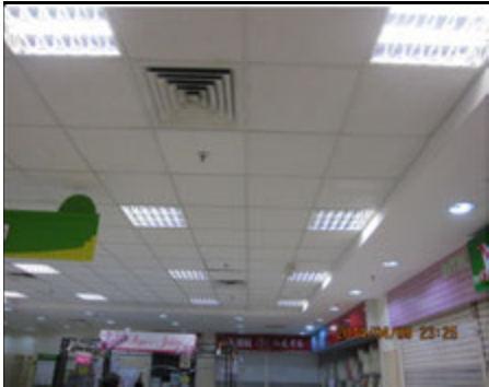
Photo 1 Complex plaster ceiling
