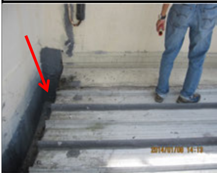
Photo 4 R C gutter
