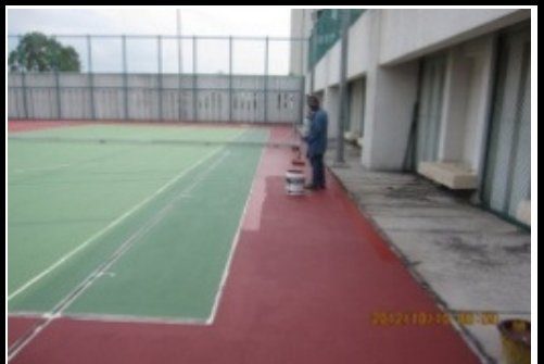
Photo 12 Another view of 2ed coat of finish acrylic textured in progress
