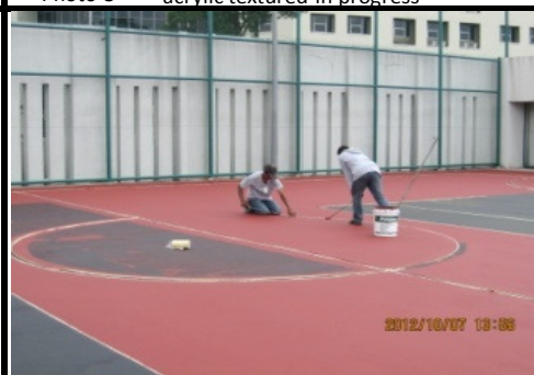
Photo 11 Another view of 1 st coat of finish acrylic textured in progress
