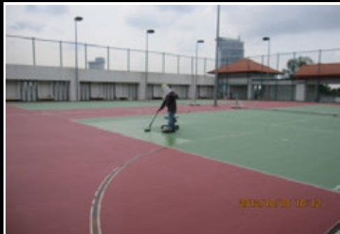
Photo 8 Another view of 3th coat of finish acrylic textured in progress
