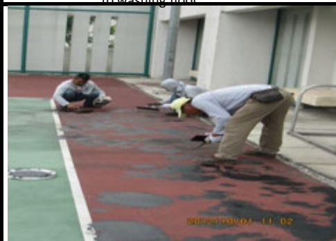
Photo 8 Another patching mix and crack filler view
