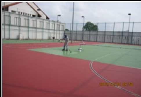
Photo 5 Another view of 2ed coat of finish acrylic textured in progress
