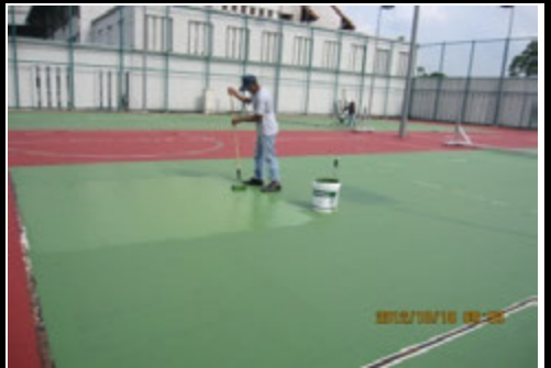
Photo 6 Another view of 2ed coat of finish acrylic textured in progress
