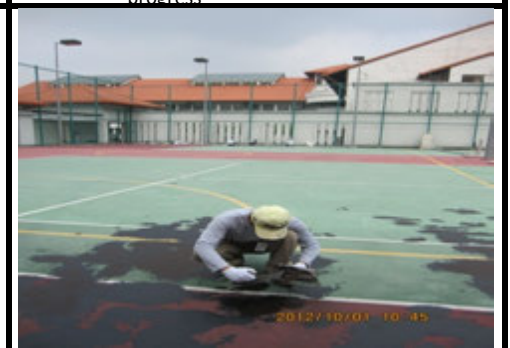
Photo 9 Another patching mix and crack filler view
