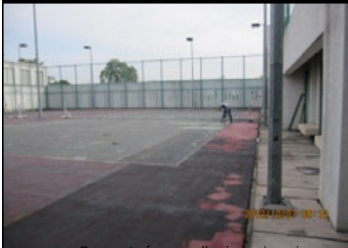
Photo 1 One coat of epoxyadhesion primer in progress
