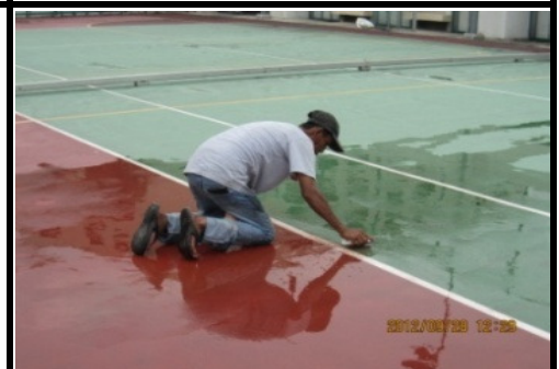
Photo 6 Brush wash to Stubborn stains in progress
