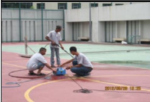
Photo 4 High pressure water jet to washing floor in progress
