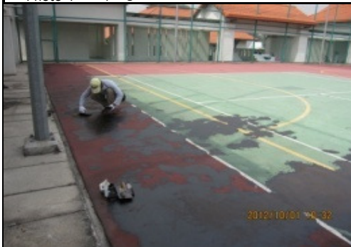
Photo 7 Patching mix and crack filler in progress
