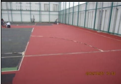
Photo 7 1 st coat of finish acrylic textured of red color in progress
