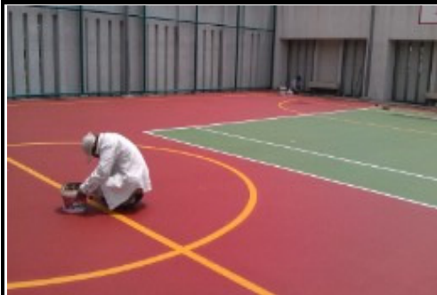
Photo 4 Paint of permanent line in progress
