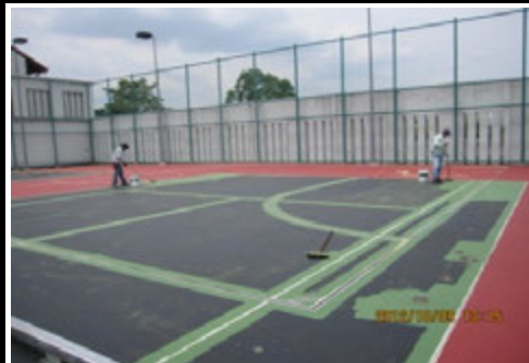
Photo 2 Another view of 1st coat of finish acrylic textured in progress
