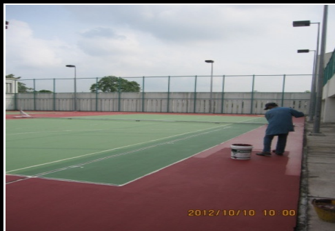
Photo 11 Another view of 2ed coat of finish acrylic textured in progress
