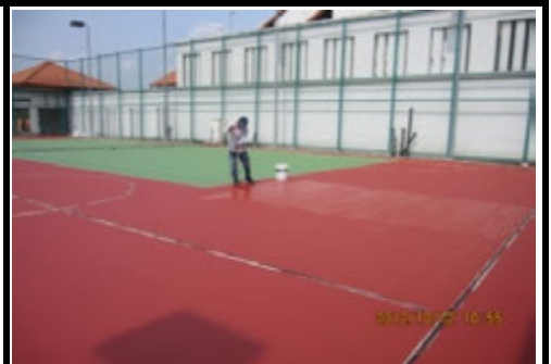
Photo 3 Another view of 3th coat of finish acrylic textured in progress
