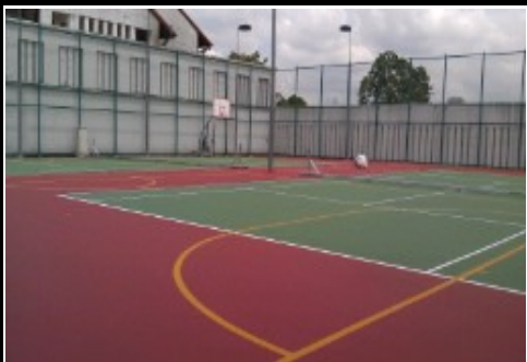
Photo 5 Another view of Paint of permanent line in progress
