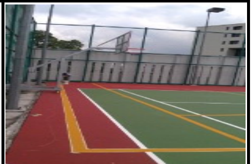
Photo 6 Another view of Paint of permanent line in progress
