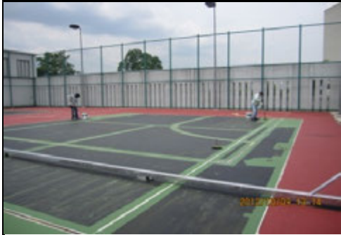
Photo 1 1st coat of finish acrylic textured of green color in progress
