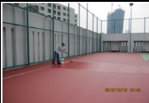
Photo 2 Another view of 3th coat of finish acrylic textured in progress
