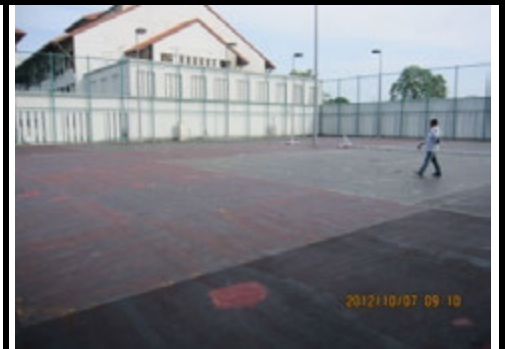
Photo 3 Another View of epoxy adhesion primer
