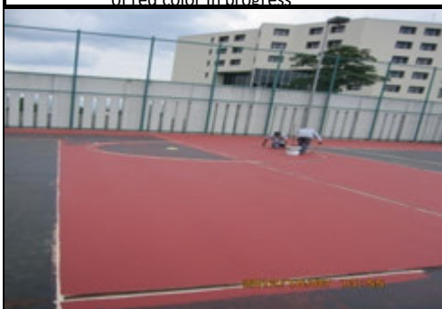
Photo 10 Another view of 1 st coat of finish acrylic textured in progress
