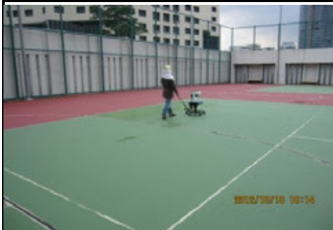
Photo 7 3th coat of finish acrylic textured of green color in progress
