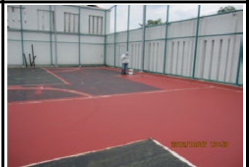
Photo 9 Another view of 1 st coat of finish acrylic textured in progress
