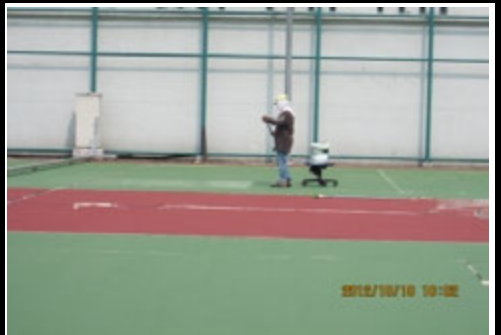
Photo 9 Another view of 3th coat of finish acrylic textured in progress
