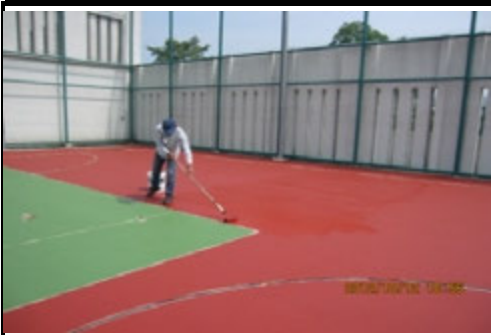
Photo 1 3th coat of finish acrylic textured of red color in progress
