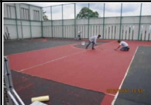
Photo 8 Another view of 1 st coat of finish acrylic textured in progress
