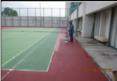
Photo 10 2ed coat of finish acrylic textured of red color in progress
