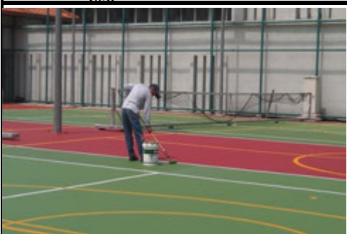
Photo 10 4th coat of finish acrylic textured of green color in progress
