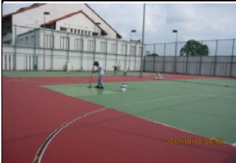
Photo 4 2ed coat of finish acrylic textured of green color in progress
