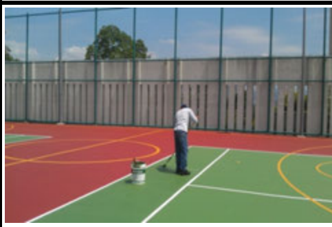
Photo 11 Another view of 4th coat of finish acrylic textured of green color in progress
