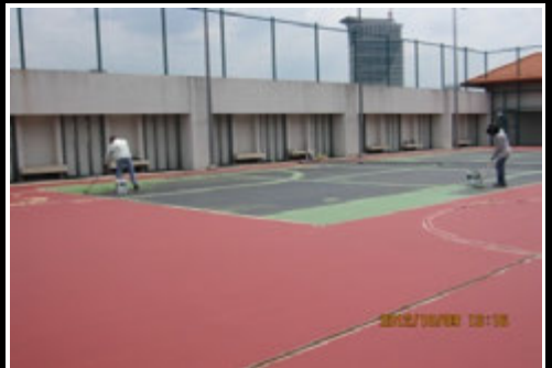
Photo 3 Another view of 1st coat of finish acrylic textured in progress
