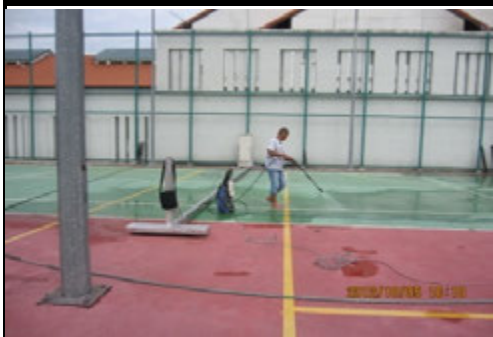
Photo 10 High pressure water jet to washing floor in progress
