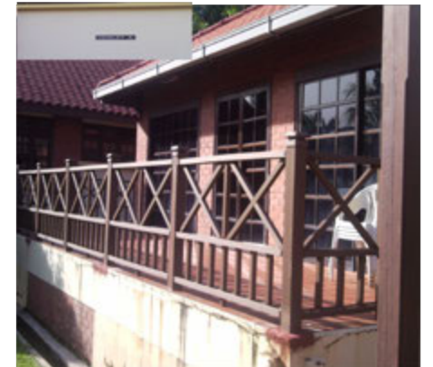
Photo 9 Chalet A rear elevation Composite Railing completed view
