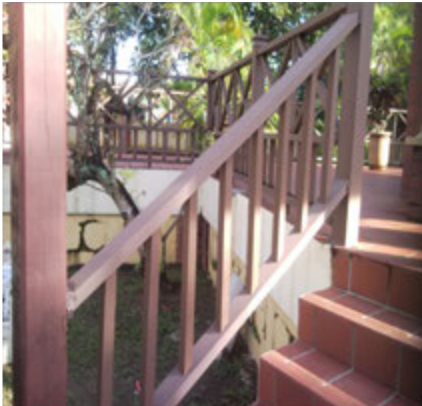
Photo 7 Another view of bungalow Gazebo Composite Railing
