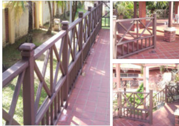
Photo 8 Bungalow Gazebo Composite Railing duly completed view
