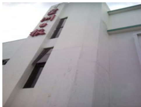
Photo 5 Staircase area view
