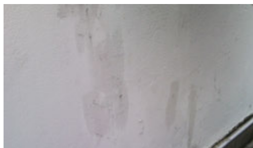
Photo 8 Defective plaster wall near toilet and staircase area view
