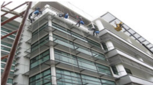
Photo 5 Commercial Abseiling cleaning system in progress...
