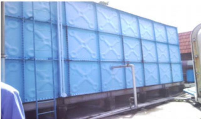
Photo 3 Side elevation of water tank view
