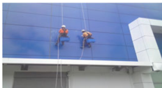
Photo 8 Hypermarket exterior window and panel cleaning system
