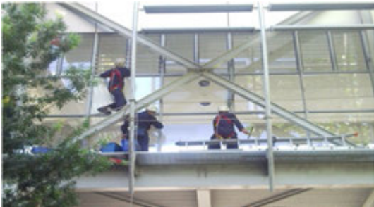
Photo 3 Hotel Cleaning System in progress...
