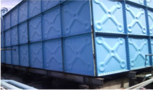
Photo 1 Front elevation of water tank view
