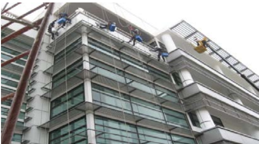
Photo 5 Commercial Abseiling cleaning system in progress...
