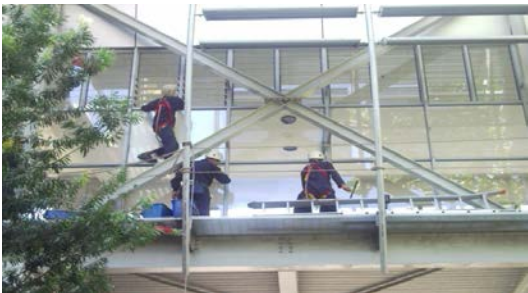
Photo 3 Hotel Cleaning System in progress...
