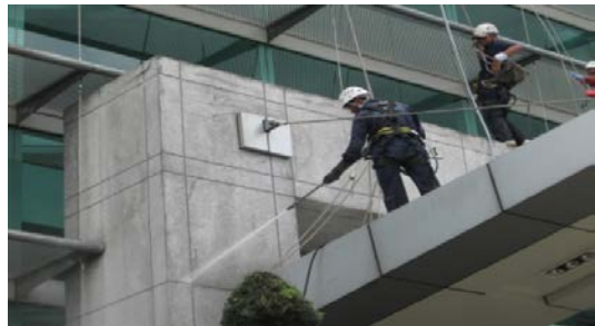
Photo 4 Commercial / Office complex Abseiling Cleaning System in progress...
