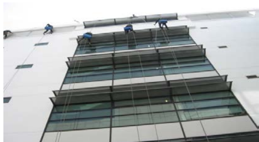
Photo 6 Glass and arocarbon abseiling cleaning system in progress...
