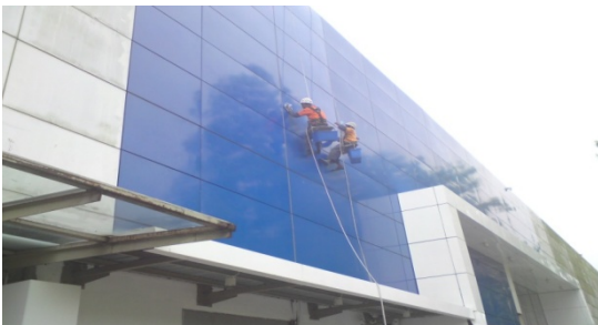
Photo 7 Hypermarket exterior abseiling cleaning system in progress...
