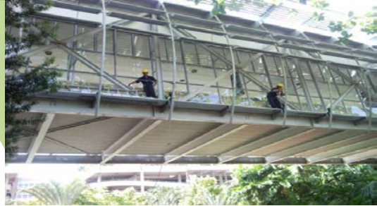
Photo 2 Another view of Hotel Abseiling cleaning system in progress...
