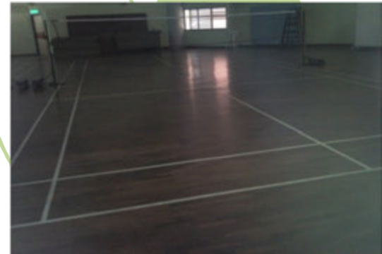
Photo 3 Existing badminton flooring general view
