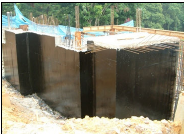
3. Completion of waterproofing membrane.
