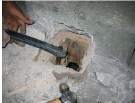
g. Remove plywood at opening soffit to do treatment
