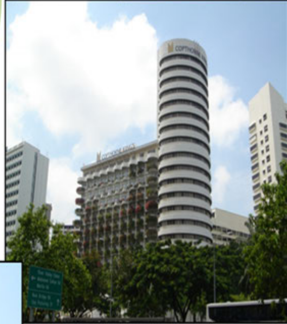
King Copthorne -360 Units ( Phase 1) -250 Units ( Phase II)
