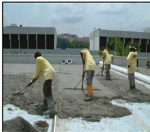
7. Casting of Gr 25 ready mix concrete panel.
