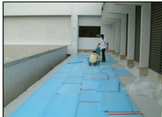
5. Laying of new 25mm insulation board and separation layer.
