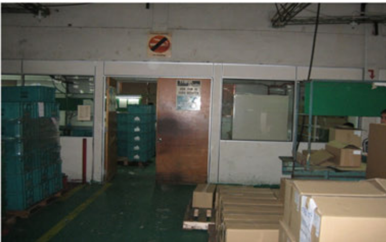
PHOTO 7 Existing inspection room required extension proposal
