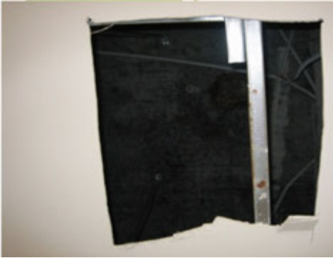
a. open Ceiling
