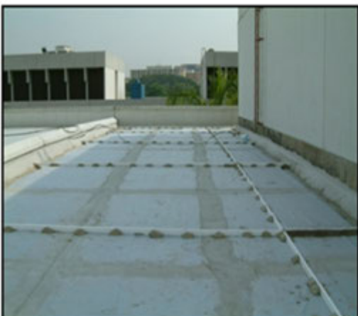
6. Constructing 12mm wide through expansion joint at every 4.5m 2 bay.
