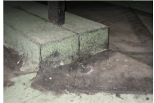
c. survey inspection at roof top to locate the opening soffit in progress....
