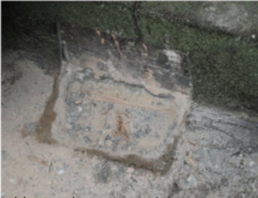
d. locate and survey to cut existing waterproofing
