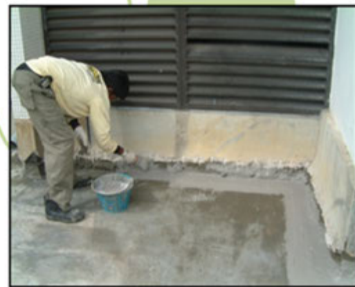
3. Patching up detailing area with cement sand mortar.
