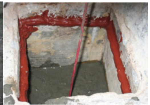
j. To apply sika sealant in progress....
