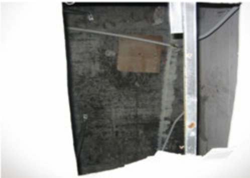
h. Insert a Plywood sealed from below opening in progress...
