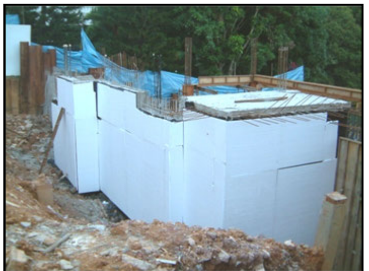
4. Installation of protection board prior backfilling.
