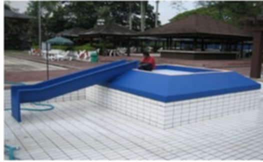
Photo 6 Painting work at pool deck in progress
