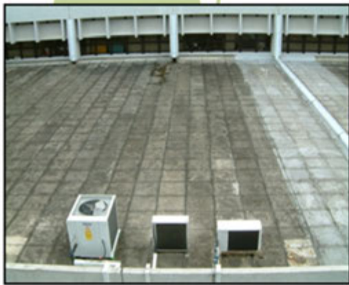
1. Existing old RC roof condition.
