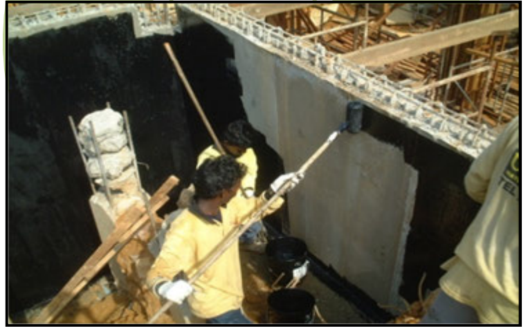
2. Application of 1 st coat waterproofing membrane.
