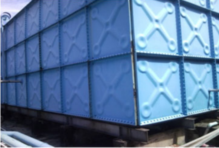
Photo 1 Front elevation of water tank view
