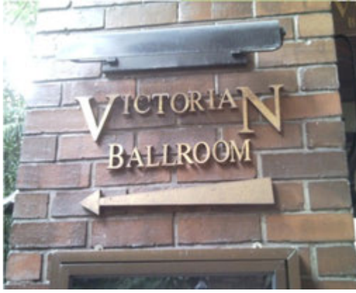
Photo 2 Victoria N Ballroom polycarbonate skylight defective view
