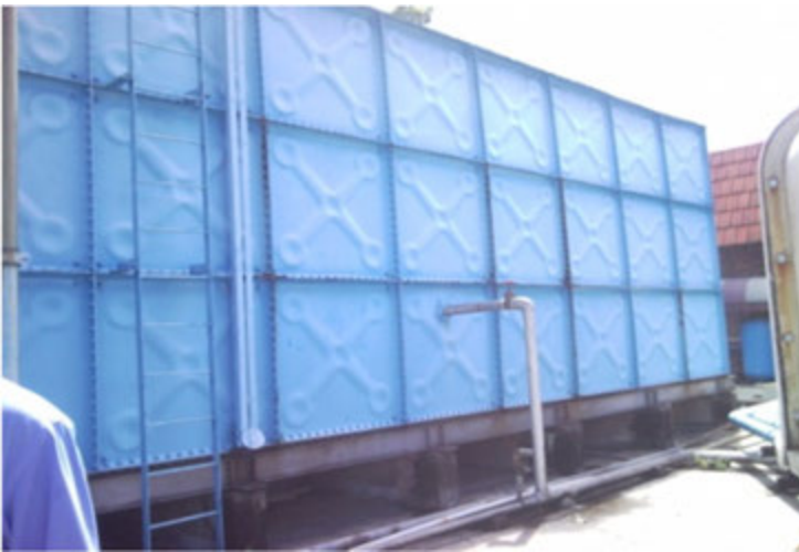
Photo 3 Side elevation of water tank view
