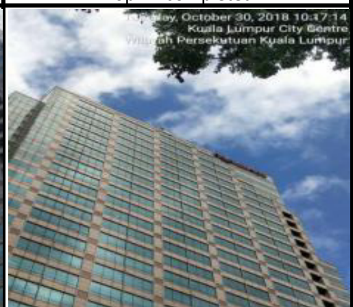
Photo 12 Stopped work due to weather
